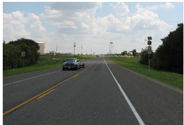
Figure 6-24. Driver's View of Approach to Study Site CV-1.
