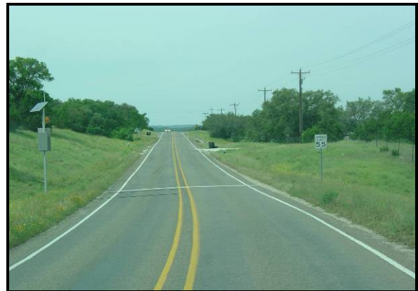
Figure 6-60. Southbound Approach to WI-1.
