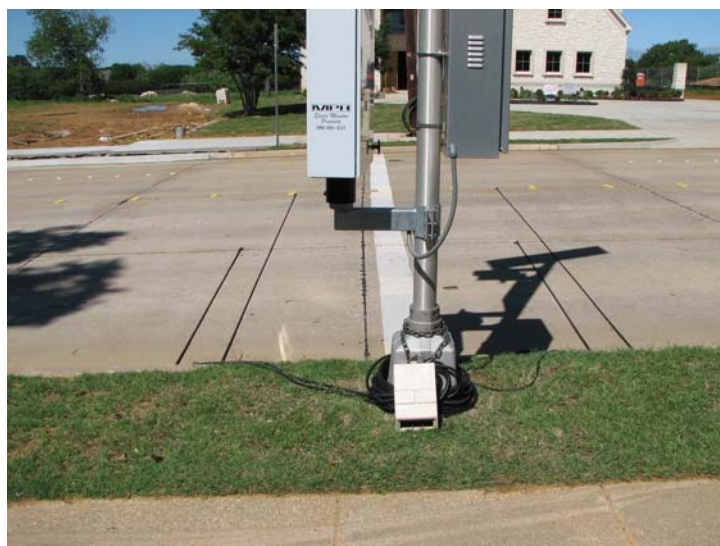
Figure 6-3. Installation of Pneumatic Tubes with Portable Counter.
