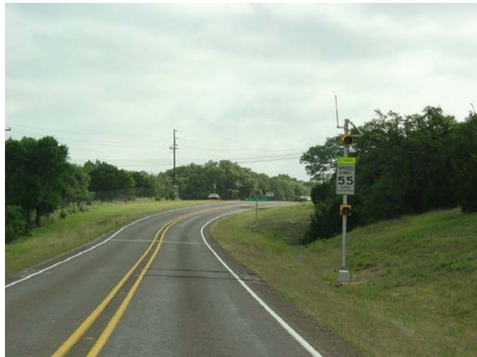
Figure 7-23. Northbound Driver's View of Buffer Zone at Site WI-1.
