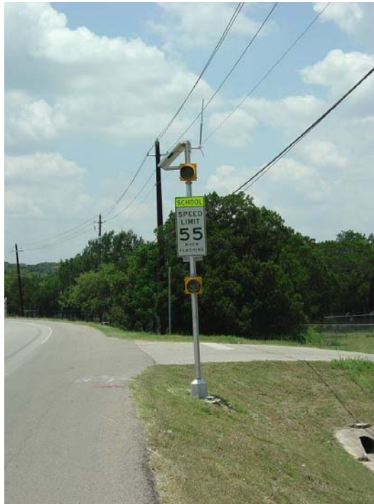
Figure 7-21. New 55-mph School Speed Limit Sign Assembly at Site AU-1.
