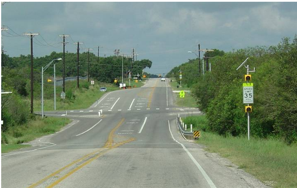
Figure 6-50. Advance Warning Sign on Eastbound Approach to SA-4.
