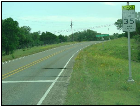
Figure 6-59. Location of Tube Detectors on Northbound Approach to WI-1.
