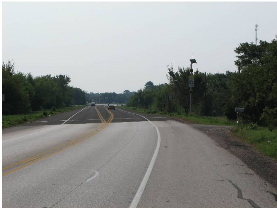
Figure 6-52. Driver's View of Approach to Study Site ST-1.
